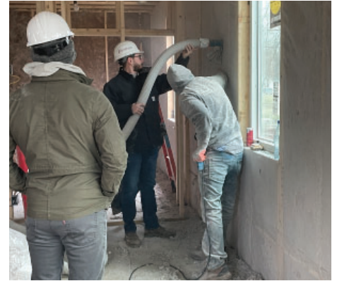
Blown-In Insulation Installation
