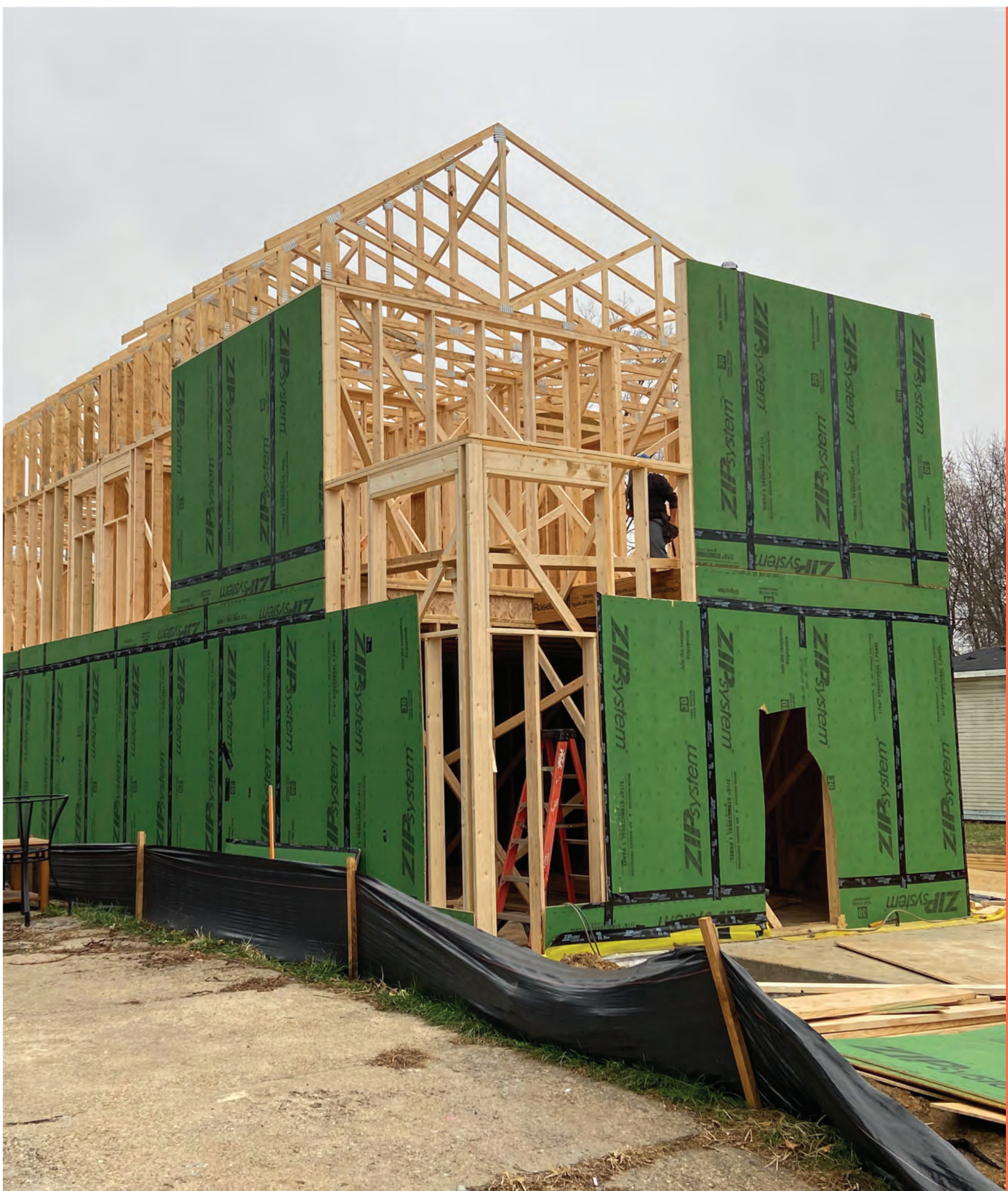
Second Floor Framing and Truss Installation
