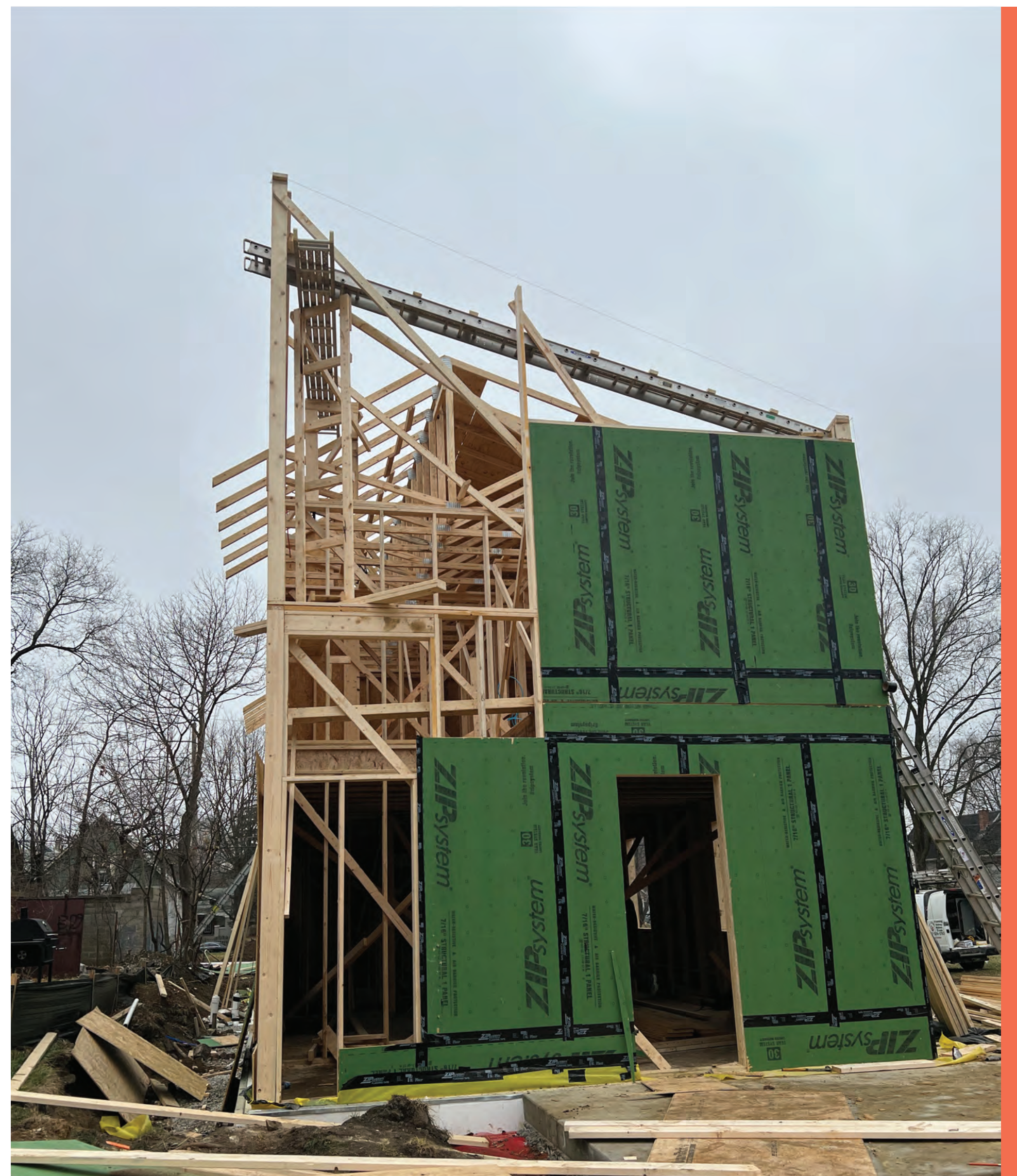
Stair Tower Rafter Installation
