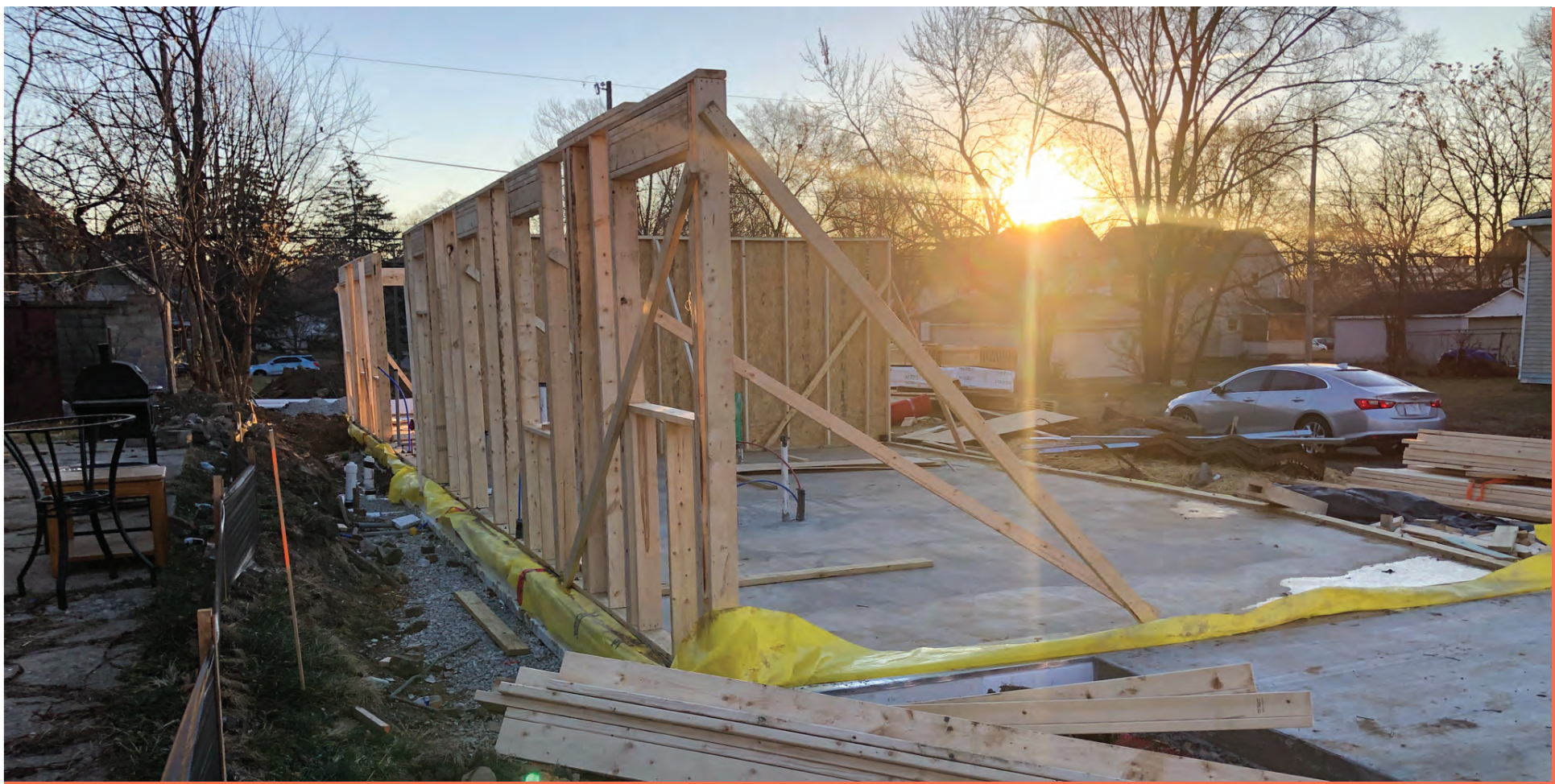
First Floor Framing
