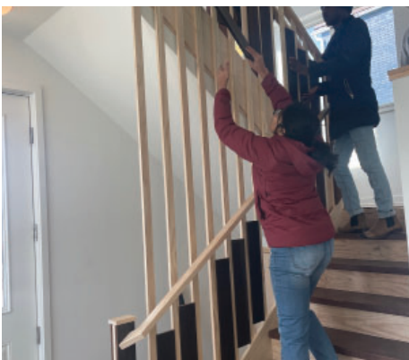
Installation Stair Railing
