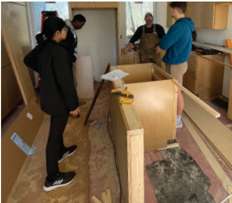
Installation of Student Built Cabinetry
