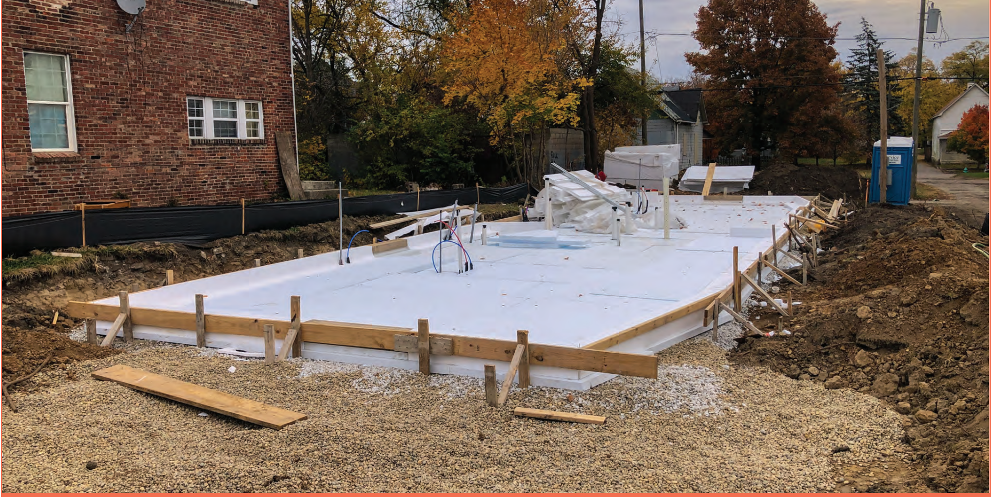
Insulation Installation
