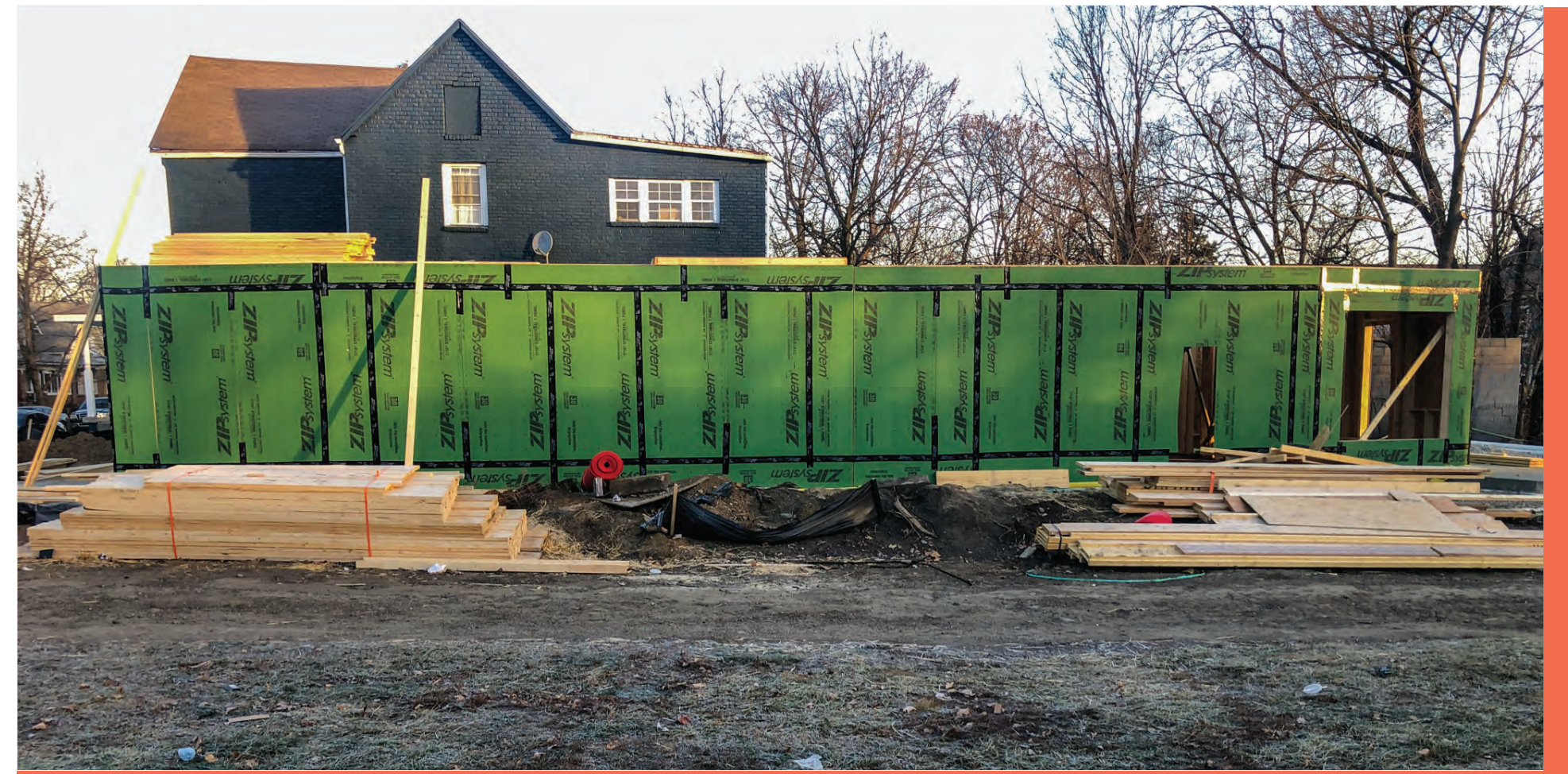
First Floor Sheathing
